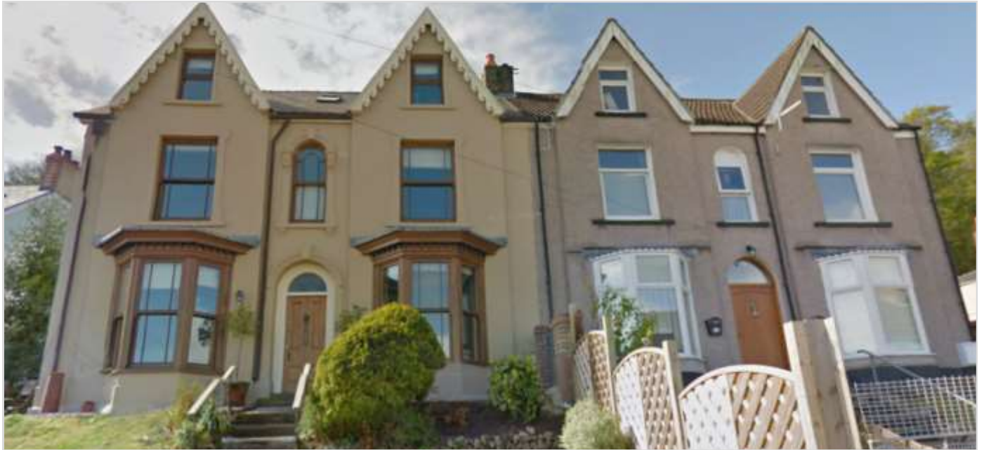
Example of a late Victorian grouping where property on the right has lost some of its heritage detail – fenestration, decorated bargeboards and ground floor bay window surround
