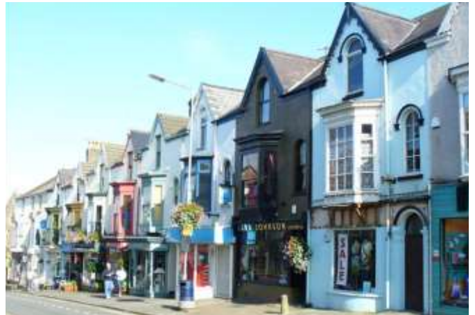
An example of the typical terrace of shops in this Character Area. The gable dormers and first floor bays create the attractive characteristics of this streetscape and limit the impact of the loss of heritage details on many buildings – chimney pots and stacks, decorated bargeboards, replacement fenestration with variety of designs, and inappropriate shopfronts and doors.
