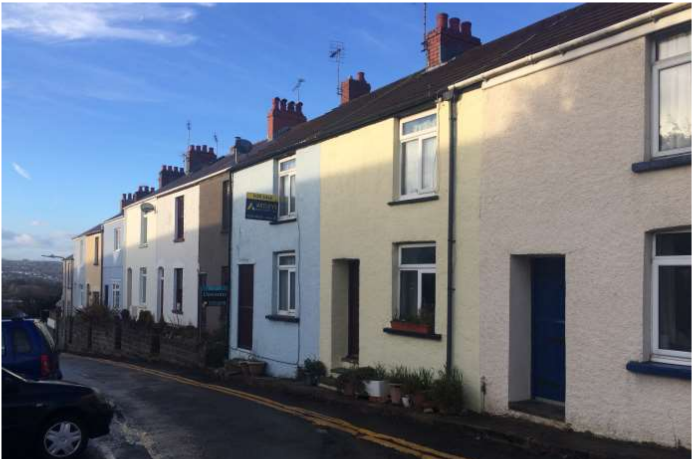
Top of Thistleboon Road showing the traditional two storey terraces stepping down the hill. Narrow roadway and problems for parking throughout the Character Area.
