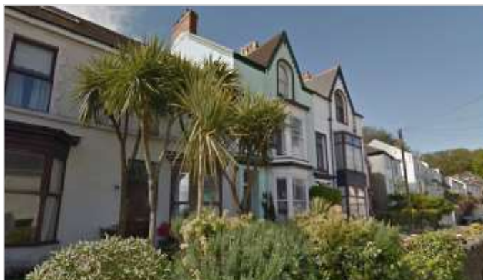
The range of Victorian and Edwardian designs of properties introduces variety and interest along the edge of the Conservation Area
