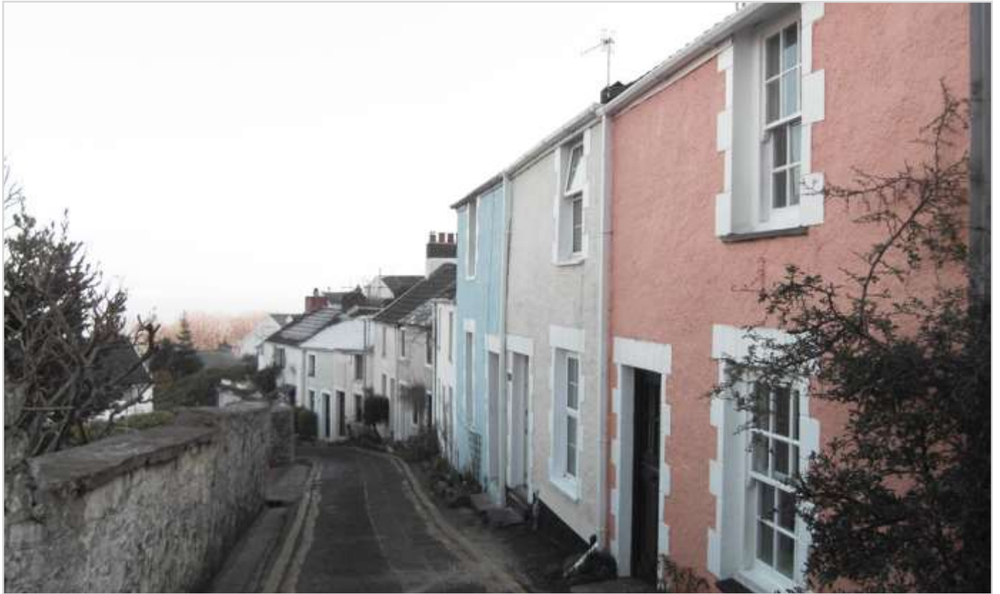
Renovated fisherman's cottages on the steep Village Lane as it climbs Mumbles Hill. The facing stone walls screens the land sloping down to the seafront but permits views over Mumbles / Swansea Bay
